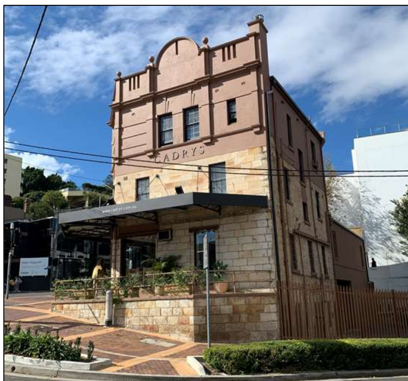
Figure 2: Cadry's Building, 133 New South Head Road, Edgecliff (viewed from the Glenmore Road to the west)
