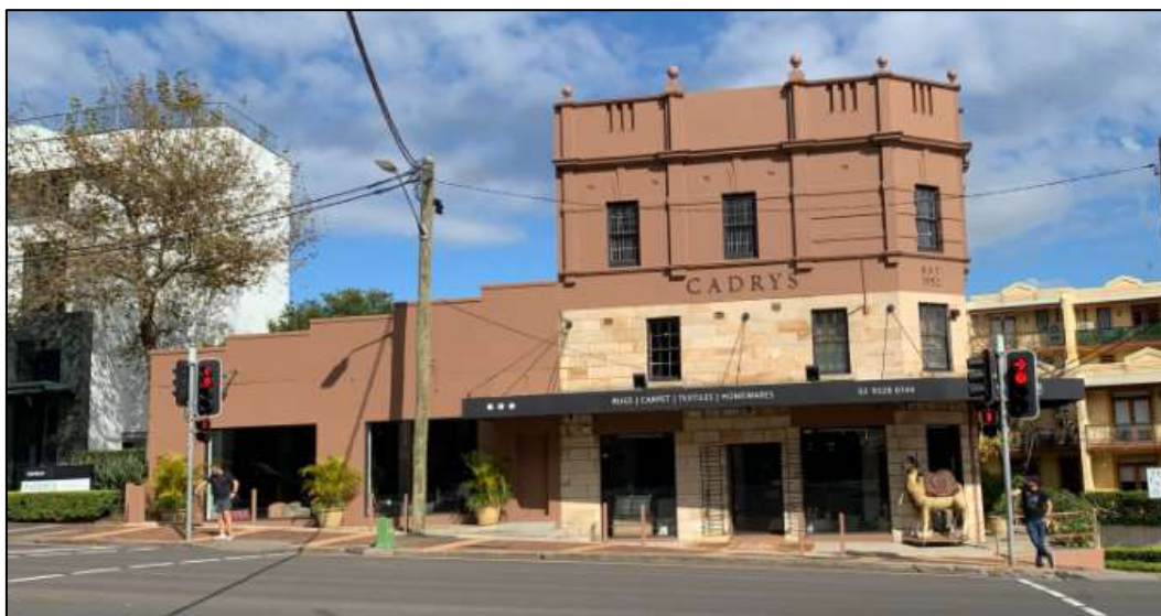
Figure 1: Cadry's Building, 133 New South Head Road, Edgecliff (viewed from the north)
