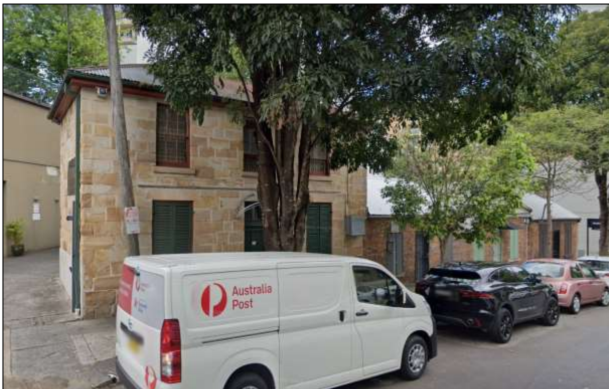
Figure 5: Two storey sandstone building at 549 Glenmore Road, Edgecliff in the left of the picture (viewed from the Glenmore Road to the west)
